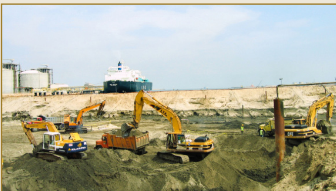
Shore protection - Methanol Terminal Project - Damietta Port, Egypt
