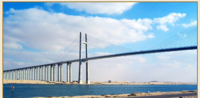
El-Salam Bridge crossing Suez Canal, Egypt
