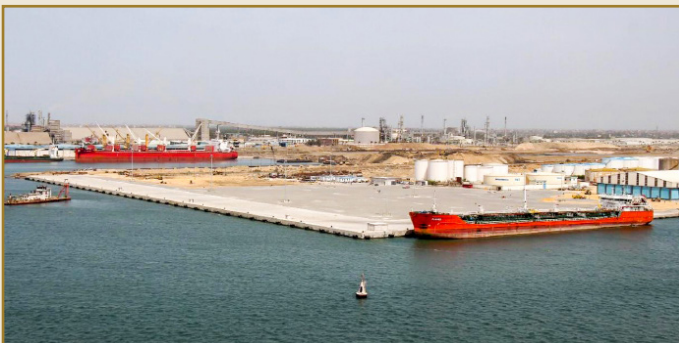
Construction of 680m berth in Damietta Port, Egypt.
