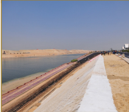
Shore Protection Works
