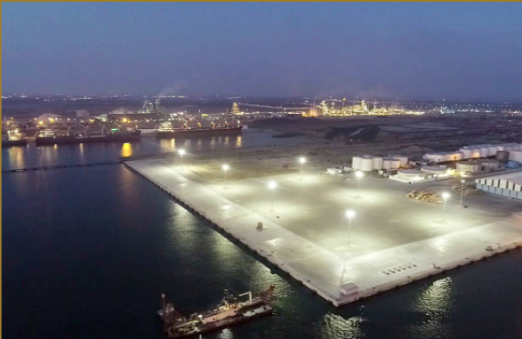
Marine Works: Quay Walls, Dredging Works, Terminal Construction, etc.
