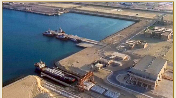
Constructing Berths 9 & 10 - Ras Al-Khair Port, Saudi Arabia
