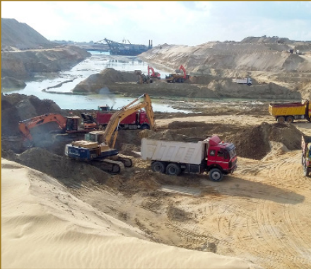
Large Scale Earthworks: Soil Improvements, Shoring & Dewatering, Excavation, Backfilling, etc.
