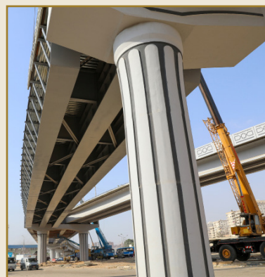
Construction of Joseph Tito Bridge length 1200 m Cairo, Egypt.
