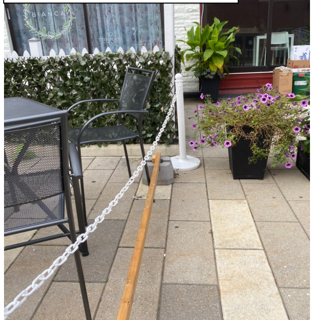
Image 3: Example of chain to post with a continuous ground level barrier.
