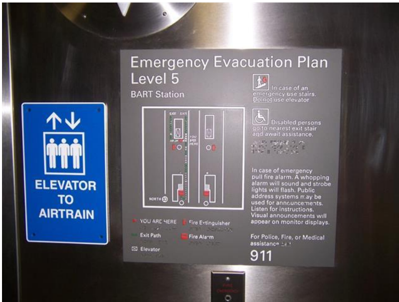
A tactile emergency evacuation plan sign. Information is presented visually and through tactile elements including a map, raised lettering, pictograms and braille.
