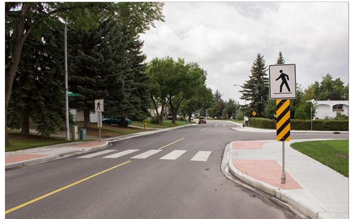
Example of a curb extension. Source: Strathcona County, 20221
