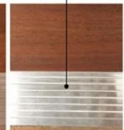
POLISHED STAINLESS STEEL TREADS PROVIDE GREATER CONTRAST AT THE TOP AND BOTTOM
