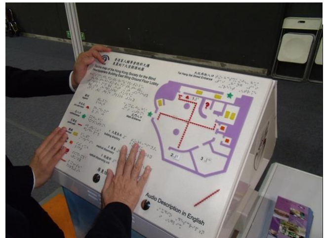
A tactile directory and map located on an inclined podium featuring braille and tactile lettering. The map incorporates colours and shape coding to identify key elements and routes. The directory also provides audio information through the push of a button.
